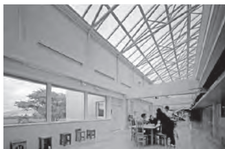
Figure 6.2.8: Renovation to upgrade a corridor into an atrium space in a glass open-ceiling style
